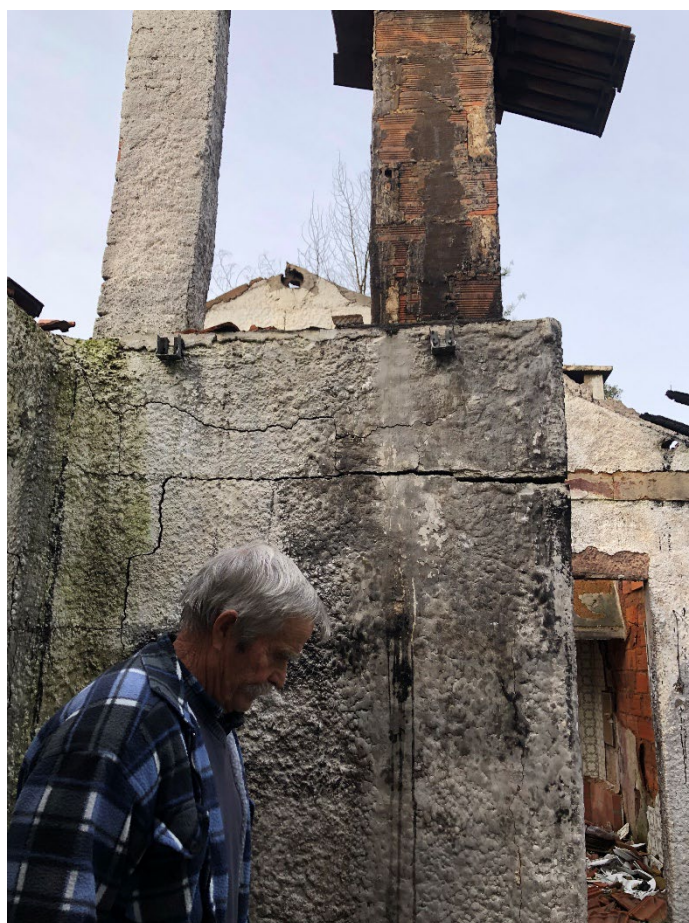
Community member in his destroyed house ©CVP
